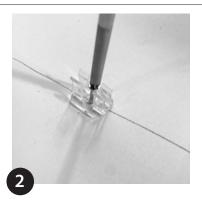
Fix clips with suitable screws.
